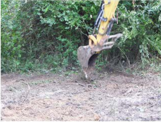
Removal of contaminated debris and soil
