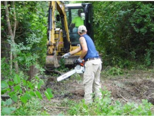
Clearing brush to accommodate cleanup
