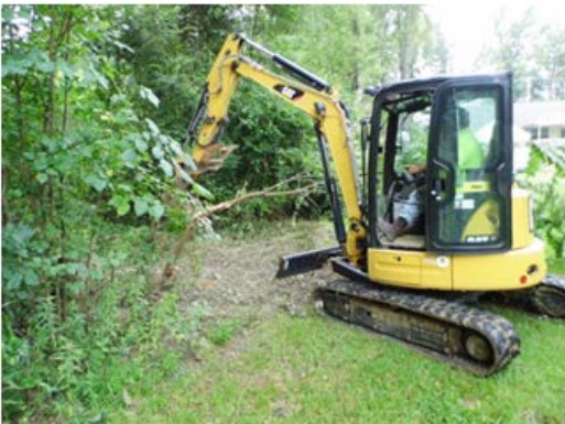
Removal of soil and debris
